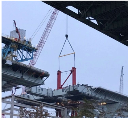
King Post Tower (12-10-2018)
