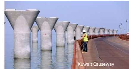
Pier Erection
